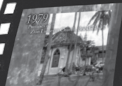
Zion Lutheran Church, Brickfields
