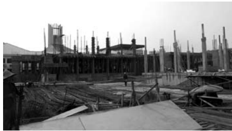
Construction in progress.
