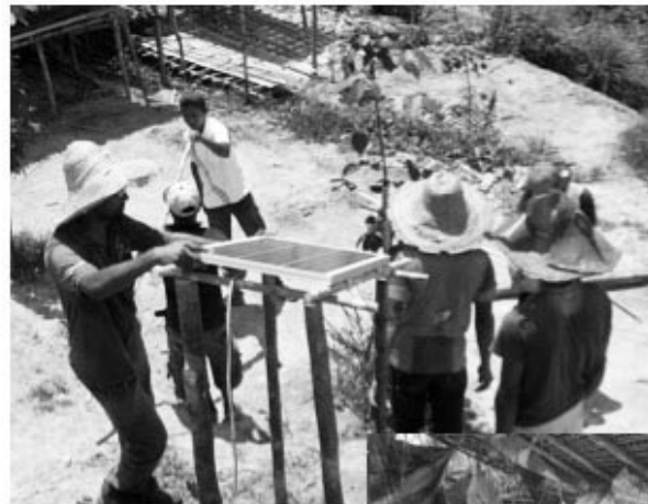
Installing solar power in a village
